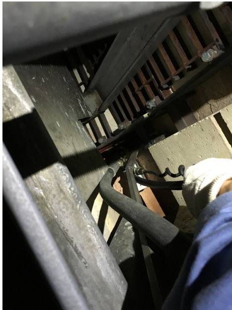
Figure 5 PaneraTech team member taking measurements on the furnace
