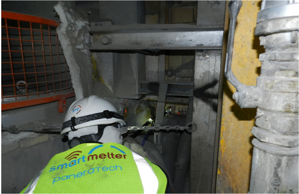
Figure 5 PaneraTech team member taking measurements on the furnace
