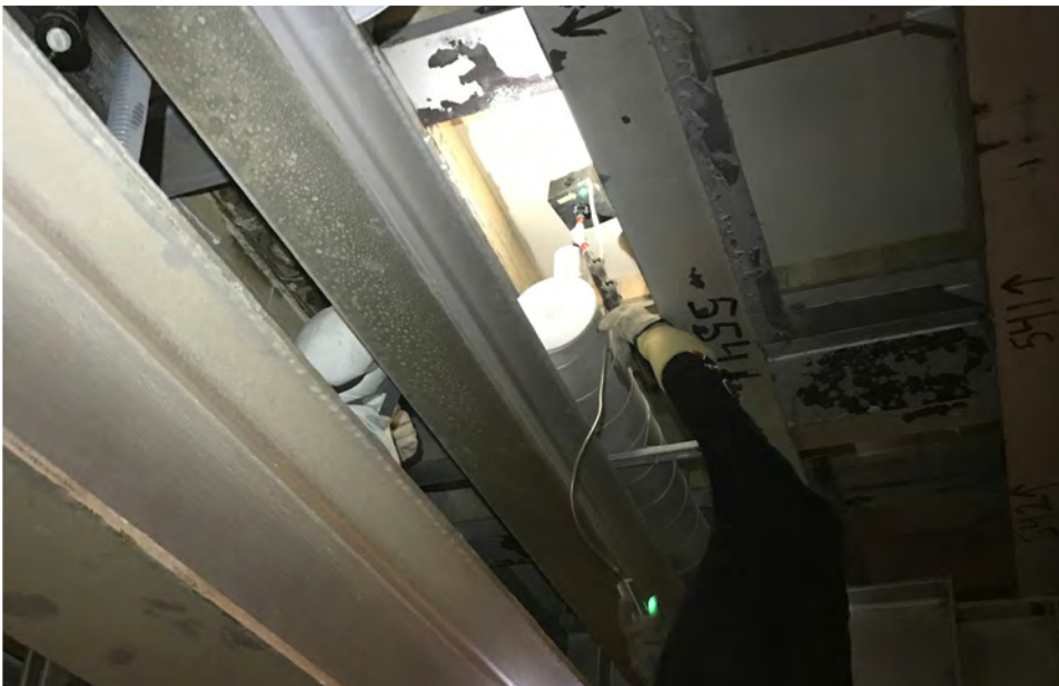
Figure 1 SmartMelter Furnace Bottom Inspection at a Float Line
